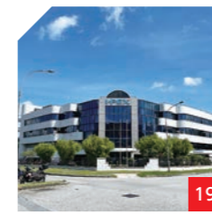
Yishun Plant, Singapore
